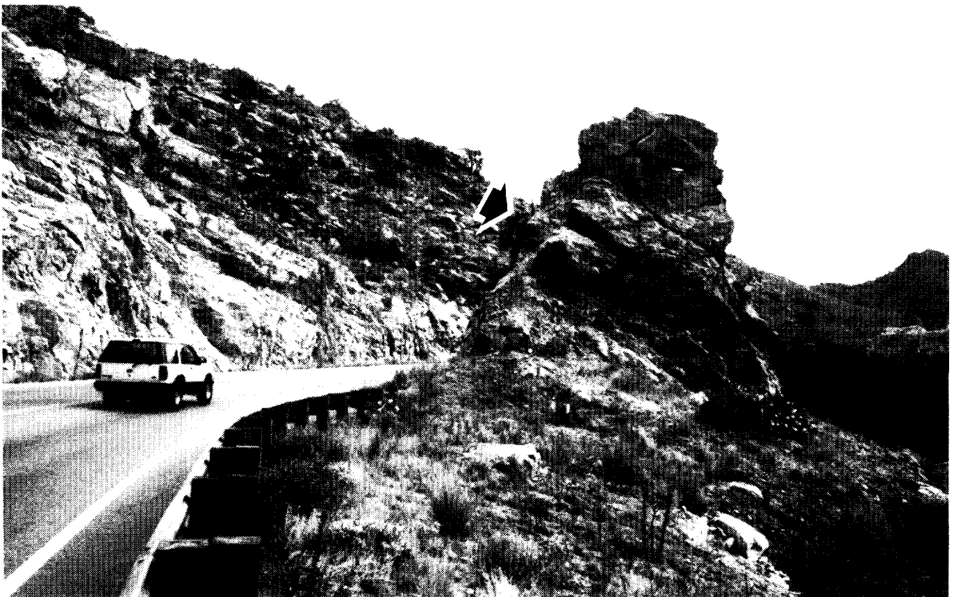
Figure B-16. Unique rock structure saved during design by alignment shift.
