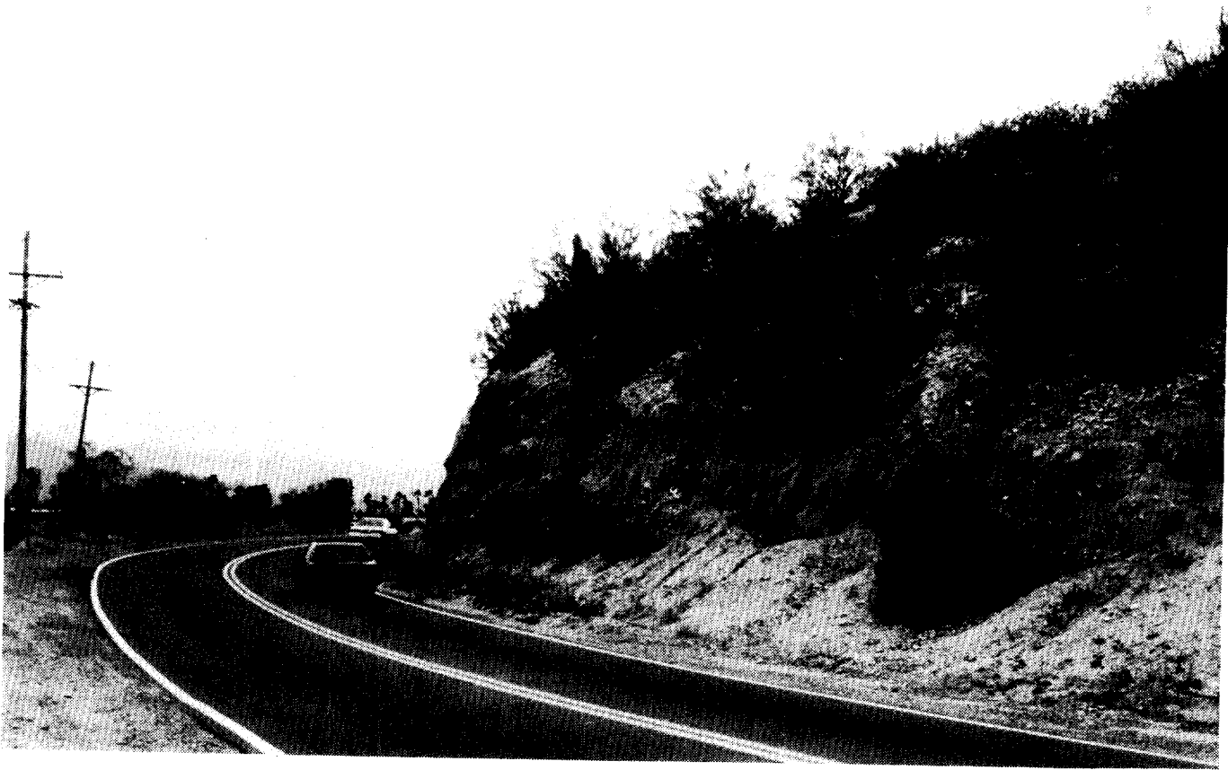
Figure B-39. Existing curve adjacent to bluff along River Road.
