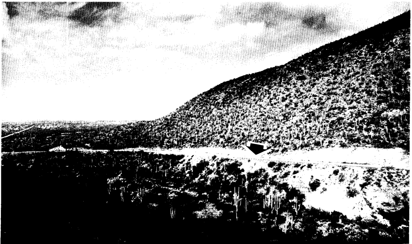
Figure B-25. Fill 3, VPL 3, 3 years after construction (see figure B-15 for comparison).
